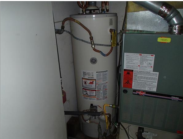
Water Heater Safety Tie Down(s) Attention
