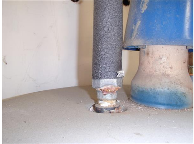
Water Heater Evidence of Encrustation Yes
